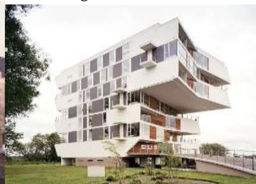
Residential building in Germany
